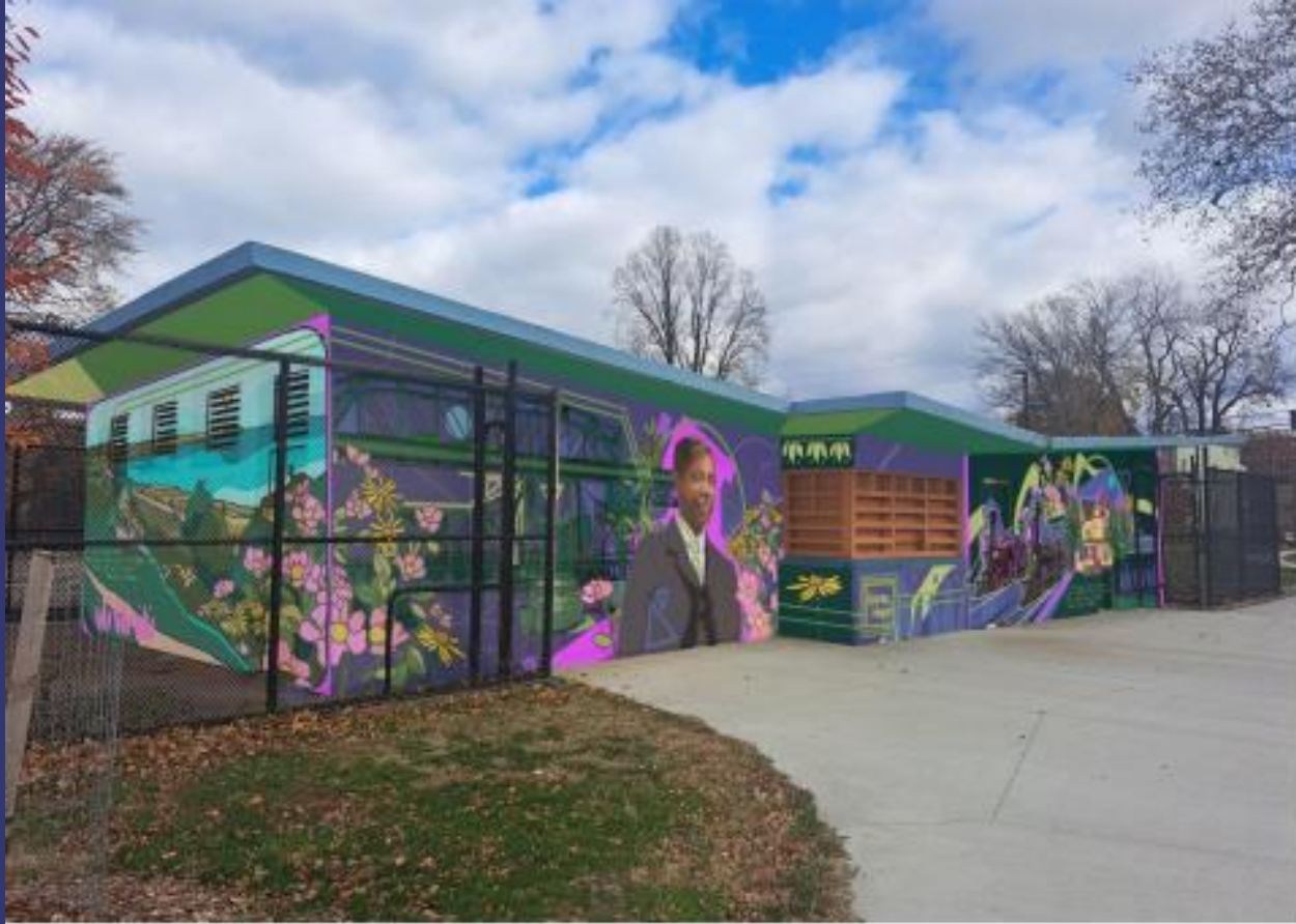
Wall facing w. 85th Street
