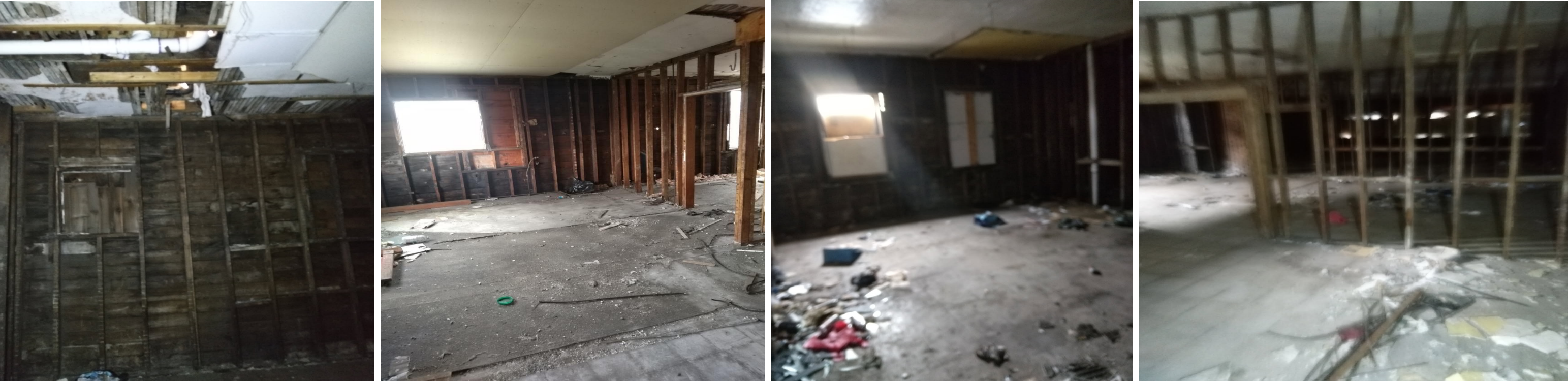
Existing Building – Interior Photos
